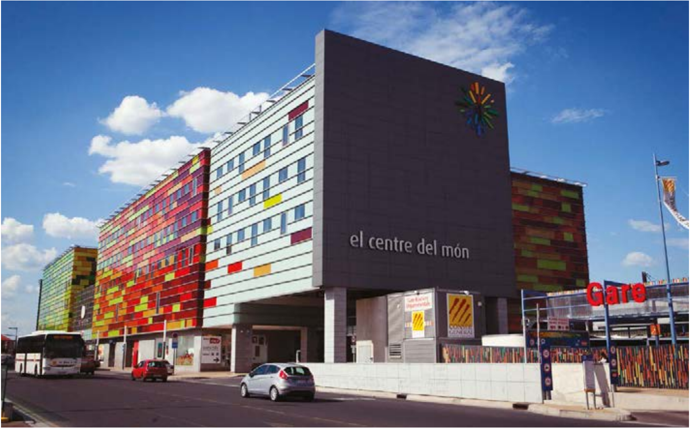
New Service Center – Perpignan, France Increasing capacity and resilience.
