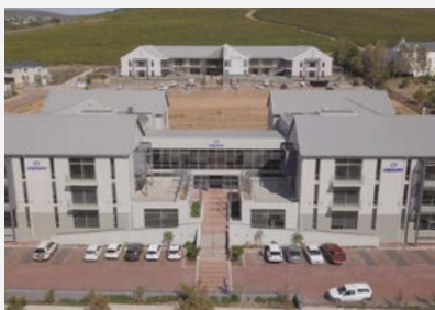
Service Center – Cape Town, South Africa The facility is the 23rd largest office to be certified by Green Building Council of South Africa in the Western Cape.
