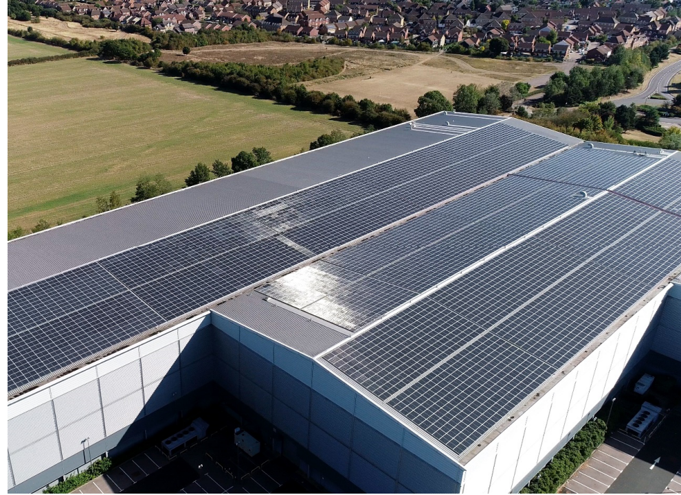
Solar panel installation – Hatfield UK
